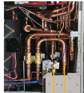
Liquid pipe Gas pipe
